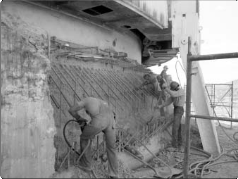
Figure 4-15. Rehabilitation of the DSS 14 hydrostatic bearing and pedestal concrete, June 1983–June 1984.
