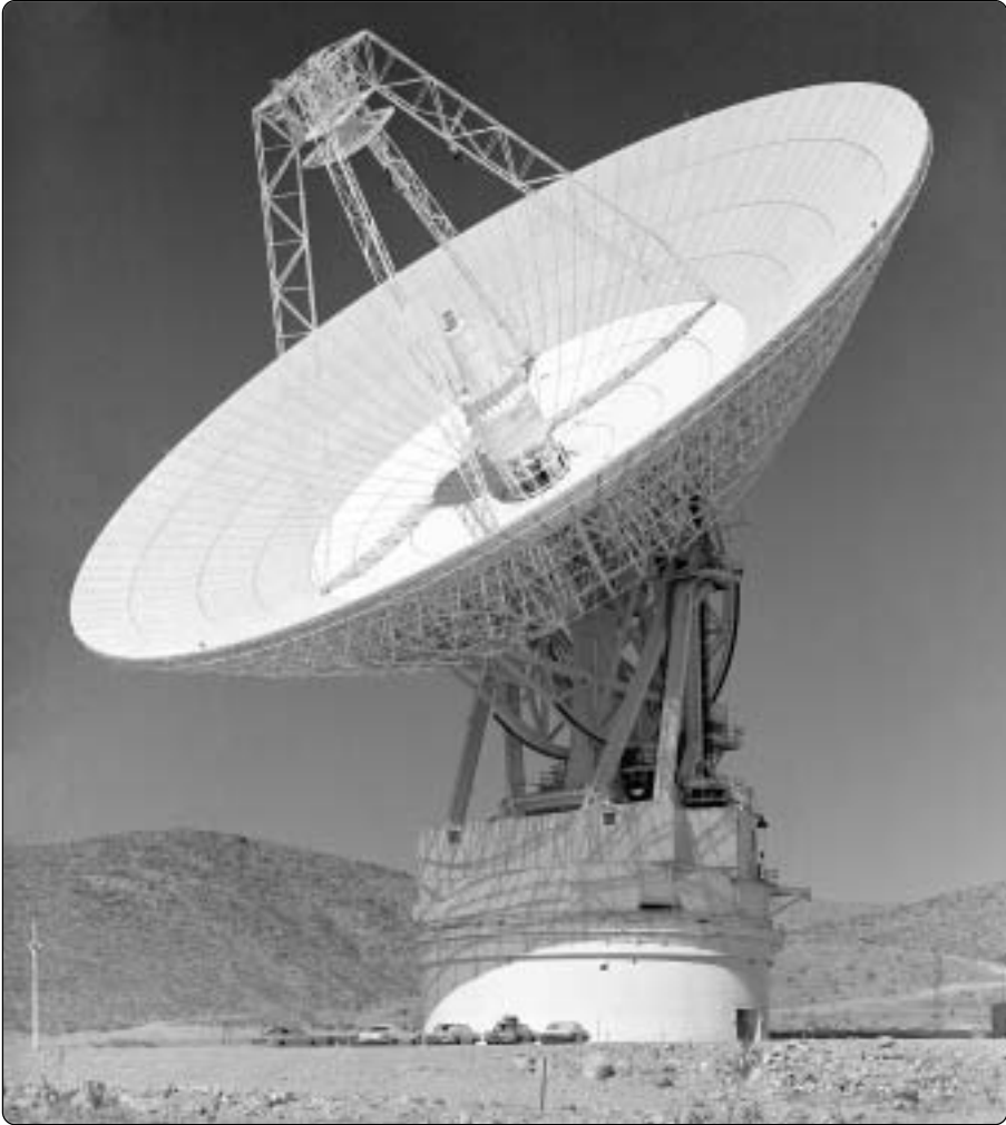
Figure 2-6. The 64-meter antenna at Goldstone, 1966. The pickup truck parked to the right side of the pedestal gives an impression of the immense size of the antenna.
