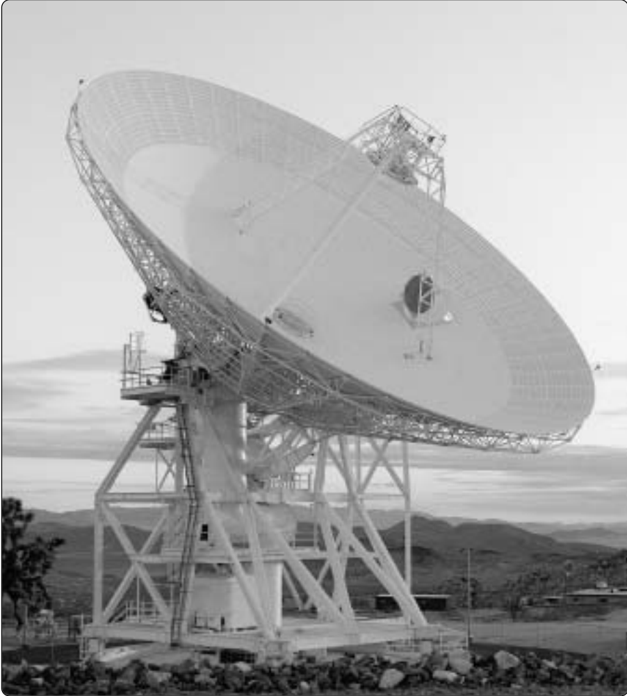
Figure 7-5. A 34-meter beam waveguide antenna at Goldstone Technology Development Site, DSS 13.
