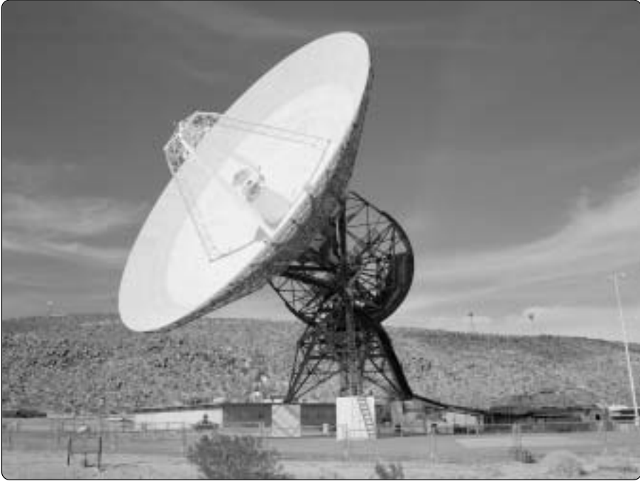
Figure 3-21. Goldstone Station, DSS 12 antenna after conversion to 34-meter, S-X-band Configuration, October 1978.
