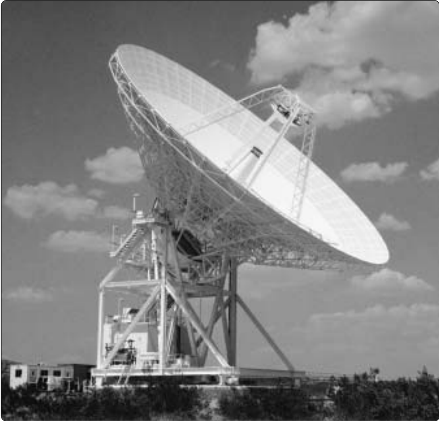
Figure 4-14. 34-meter high-efficiency (HEF) antenna: DSS 15, Goldstone.
