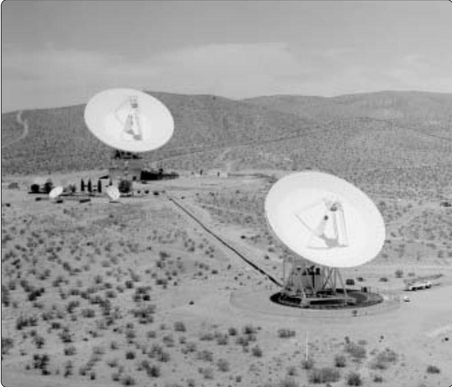
Figure 7-3. The quasi-parabolic 34-m high-efficiency (HEF) antenna, DSS 15.
