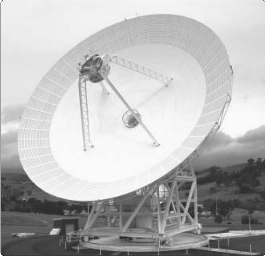
Figure 5-36. DSS 34 BWG antenna at the Canberra Deep Space Communications Complex, Australia, 1996.
