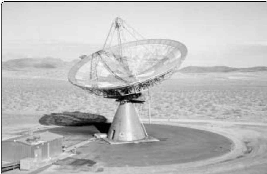
Figure 1-5. Az-El transmitting antenna for the Echo Balloon Experiment, Goldstone, 1960. The antenna was constructed between July and December 1959, and the complete station became operational in July 1960.
