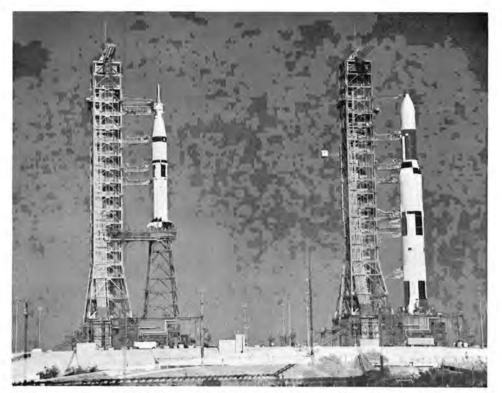
A double exposure of the Skylab 1 and Skylab 2 space vehicles, actually 2.4 km apart on their launch pads. The unmanned Skylab 1, at the right, was launched 14 May 1973 on the last Saturn V to be flown. *Skylab 2*, with the smaller Saturn IB perched on the "barstool" support tower, lofted astronauts to rendezvous with *Skylab 1* on 25 May 1973.
