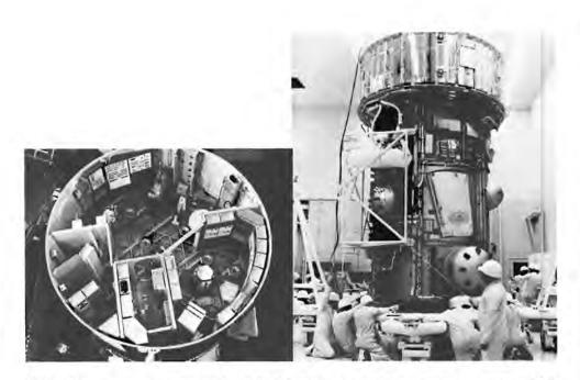
Left, the crew quarters area of the Skylab Orbital Workshop training model, which had been shipped from MSFC to MSC to be used for Skylab mission crew in flight simulation exercises. Right, the airlock module flight article is shown in a clean room at the McDonnell Douglas facility at St. Louis before being mated with the multiple docking adapter. The airlock module provided a pressurized passageway between the multiple docking adapter and the Orbital Workshop.
