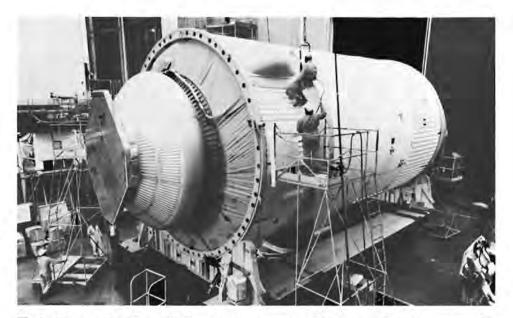
Technicians at McDonnell Douglas Astronautics, Huntington Beach, prepare the Skylab Workshop test vehicle for shipment to MSC and MSFC to undergo design verification tests. The test article was subjected to acoustic, vibration, and static forces comparable to those that would be encountered during launch and orbit.
