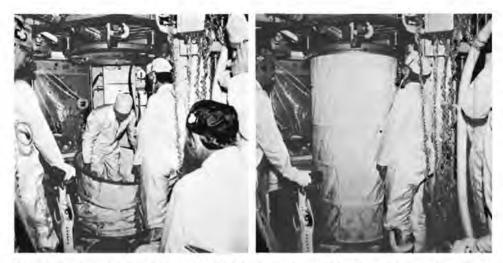
Provisions were made so that each Skylab astronaut could take a shower every week. MSFC designed and built a shower assembly to be stored as a compact unit in the crew quarters area of the workshop. At the left is a demonstration of the manner in which an astronaut would step inside a ring mounted on the floor and raise the 109-cm-diameter hoop to form the shower area. The extended curtain is then attached to the ceiling (right), and the shower is ready for use.
