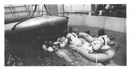
Skylab 3 crewmen (left to right) Alan L. Bean, Owen K. Garriott, and Jack R. Lousma during egress training at MSFC before their liftoff. This operation was an alternate recovery plan in case of rough seas and the command module's floating in the upside-down position.
