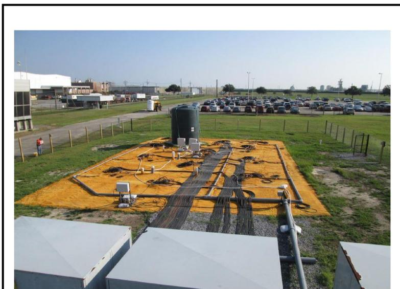
Remediation of contamination in the groundwater at MAF. Electrical current is applied through electrodes driven into the ground and the contaminated soils and groundwater are heated. The volatilized contaminants are removed through vacuum extraction.
