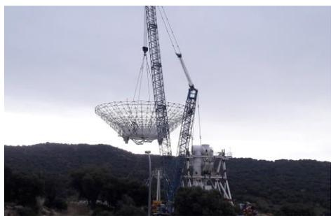
**The skeleton of the antenna reflector of the Deep Space Station - 56 (DSS-56) was lifted on its pedestal in November 2018.**
