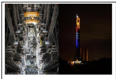
At left, a view of High Bay 3 inside the KSC Vertical Assembly Building (VAB) showing platform halves installed. Note in the background the Mobile Launch Tower (MLT) undergoing preliminary fit-checks assessment. On the right is a view of the MLT undergoing final preparation just prior to being transported by the Crawler to LC-39B and VAB.
