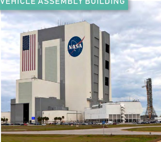
The iconic VAB at NASA's Kennedy Space Center in Florida, to the right a crane positioning the Orion crew access arm for assembly to the mobile launcher. Photo Credit: NASA/Bill White
