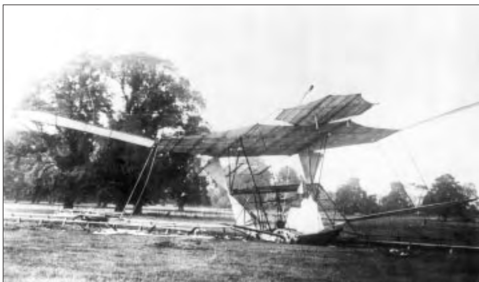
Maxim's huge four-ton biplane, with its eighteen-foot propeller, sits on its track ready for flight testing (unsuccessful) in 1894. Ultimately the monster rose slightly from its guardrails, but only after traveling some 600 feet down the track. It possessed no truly redeemable features and represented, in its two very efficient steam engines, a brute force approach to getting an airplane aloft. SI Negative A-212-A
