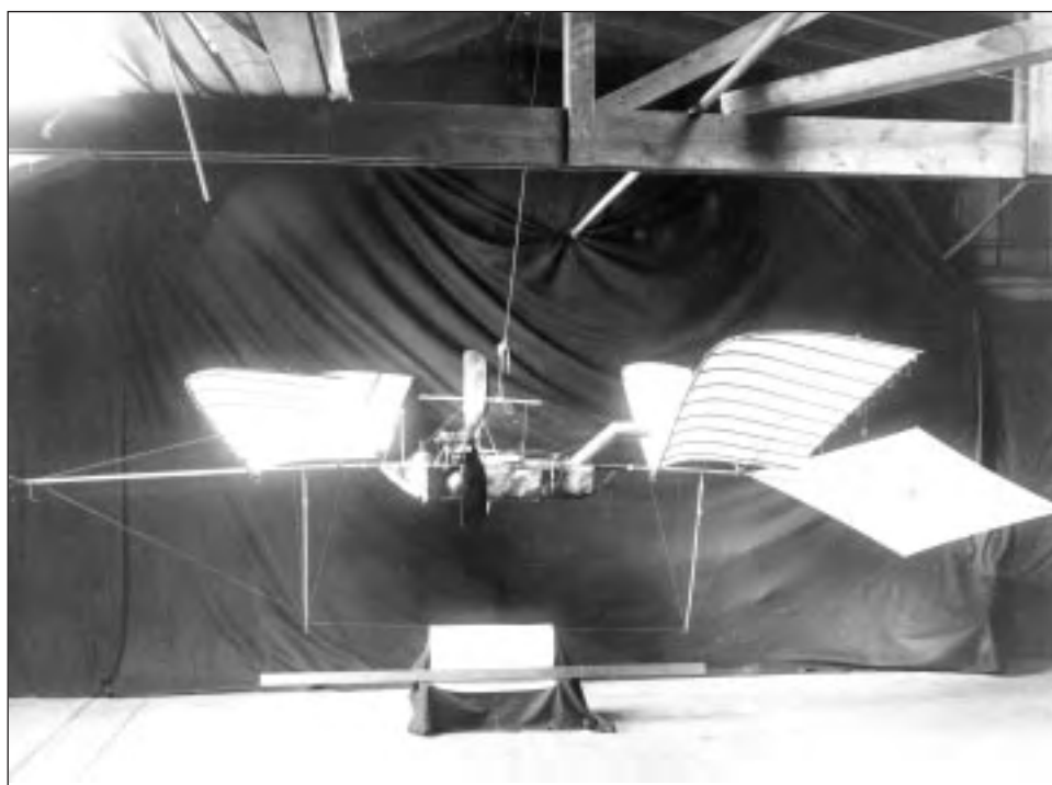
Although he ultimately failed in his effort to build a successful man-carrying airplane, one should not minimize Professor Samuel P. Langley's many contributions to aerodynamic understanding, especially those embodied in the flights of his large steam-powered models in 1896. In this photograph from December 1895, Langley's Aerodrome No. 6 (which evolved from No. 4 ) had not yet matured into its final configuration. SI Negative No. A-2854-J
