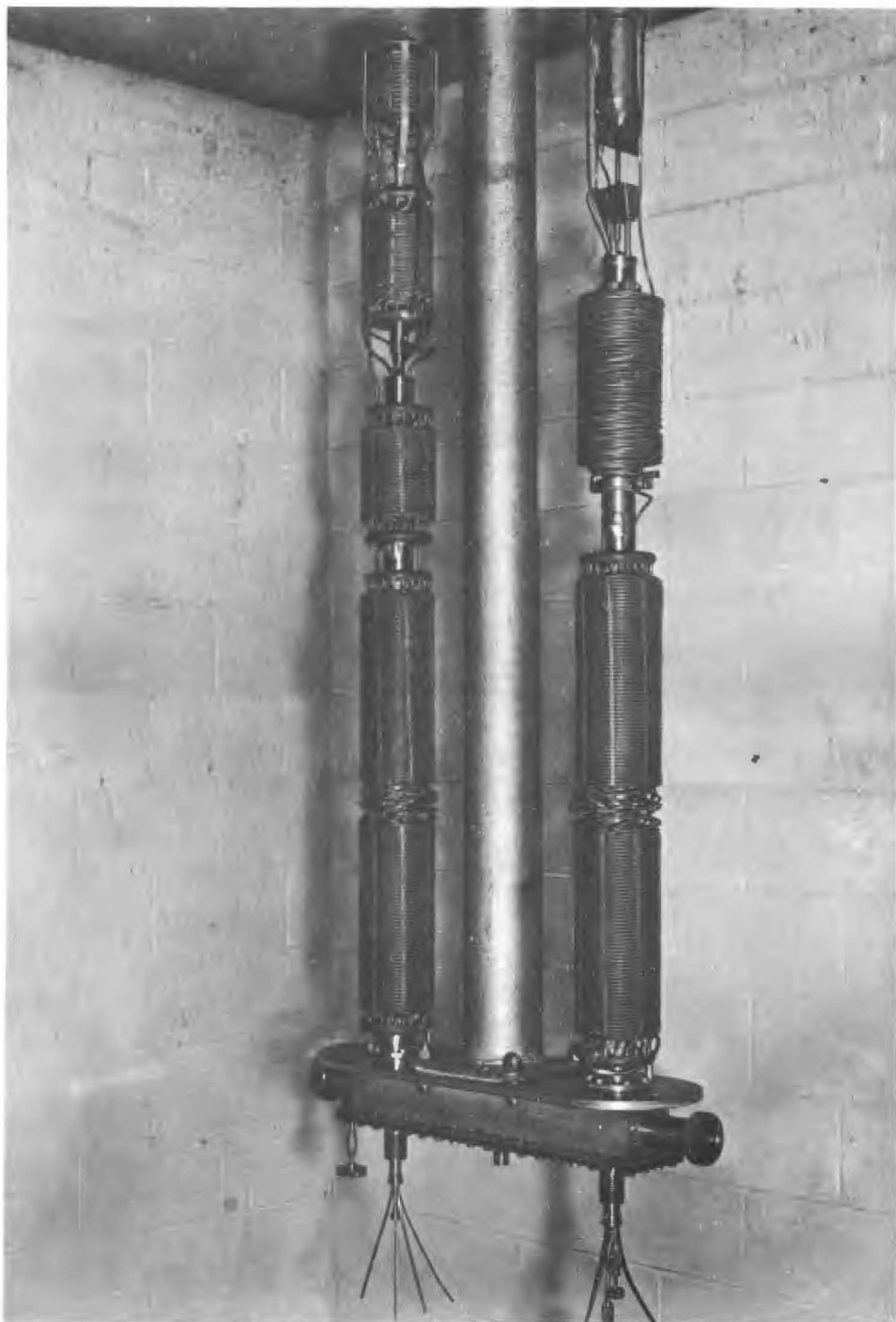
Fig. 2. The several heat exchangers (shell removed) of H. L. Johnston's hydrogen liquefier, ca. 1946. (Courtesy of W. V. Johnston.)
