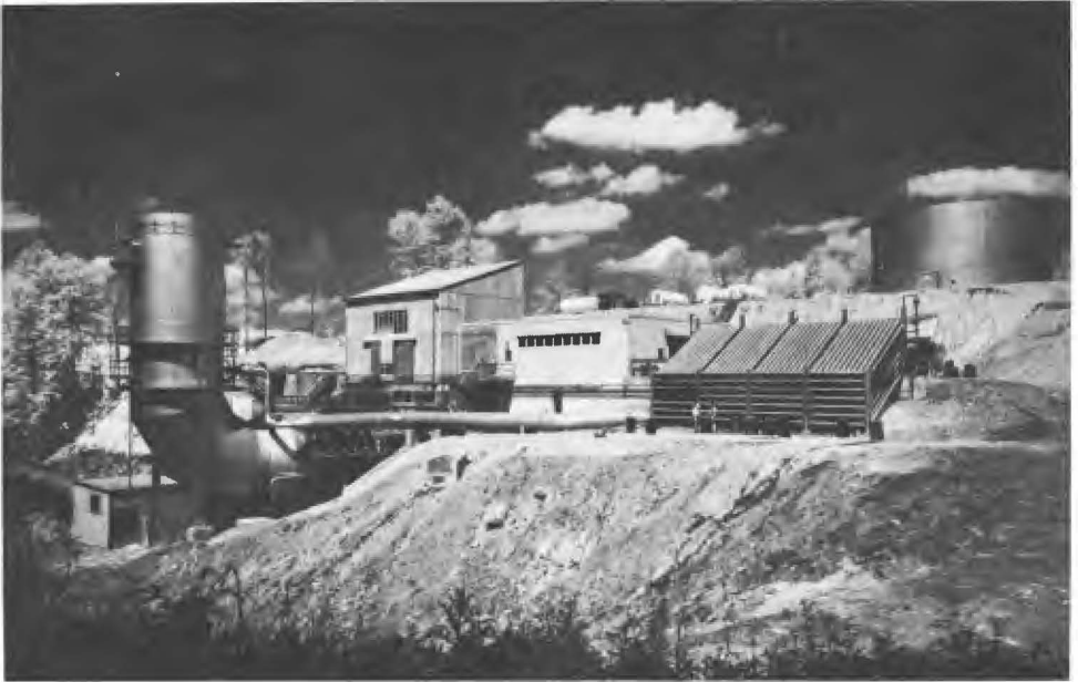
Fig. 15. The NACA-Lewis high-energy rocket propellant test facility, placed into operation in 1957. The building with the slanted roof is the test cell. The large horizontal duct with vertical stack is the exhaust-gas scrubber and silencer. The two men are in front of racks of high-pressure cylinders of helium used for pressurization. On the far right is the water storage tank and on the far left is the water detention tank and treatment system.
