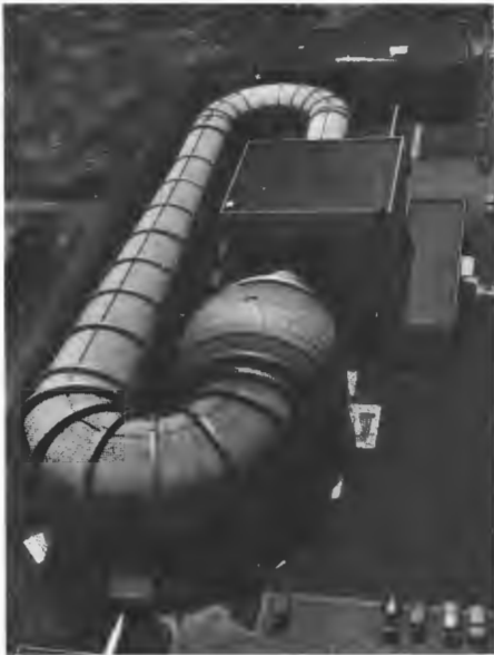
Completed 12-foot tunnel, May 27, 1946.
