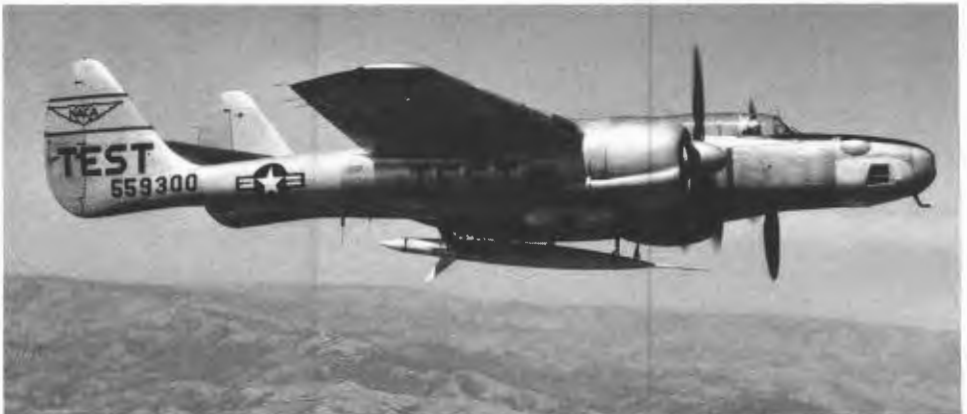
Northrop P-61 airplane used in drop-test technique.
