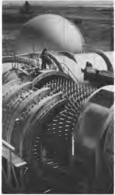
The 6- by 6-foot tunnel compressor, one of the early applications of multistage axial-flow compressors to wind-tunnel-air propulsion.
