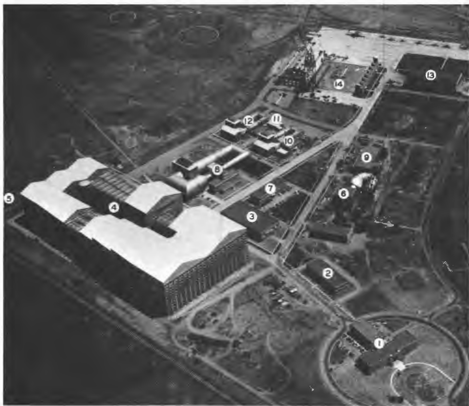
Aerial view of Ames Aeronautical Laboratory on July 3, 1945, at the end of World War II. (1) Administration building, (2) Science laboratory, (3) Technical service building, (4) 40- by 80-foot wind tunnel, (5) Substation, (6) 12-foot pressure wind tunnel, (7) Utilities building, (8) 16-foot high-speed wind tunnel, (9) 1- by 3-foot supersonic wind tunnels, (10) 7- by 10-foot wind tunnel no. 1, (11) Model finishing shop, (12) 7- by 10-foot wind tunnel no. 2, (13) Flight research laboratory, and (14) Airplane hangar and shop.
