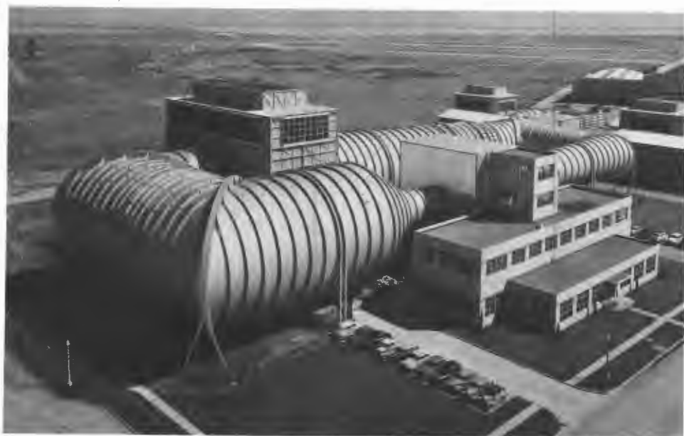
Above: 16-foot wind tunnel. Below: Ames Aeronautical Laboratory on June 10, 1942. Completed buildings include the flight research laboratory, science laboratory (near circle), technical service building, utilities building, and three wind tunnels. Electric substation and outline of 40- by 80-foot tunnel can be seen.
