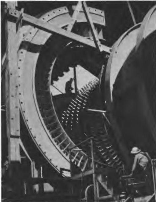
11-stage compressor of the Unitary Plan wind tunnel.
