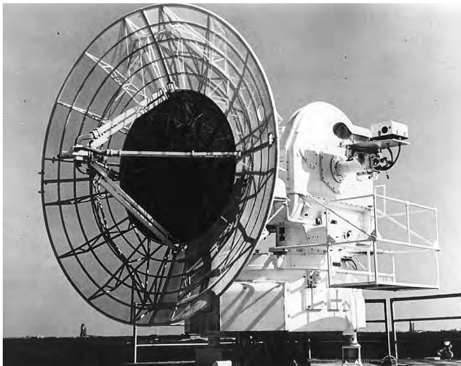
The RCA FPS-16 radar has been widely used at missile ranges since the 1950s. It is a transportable, Single-Object Tracking Radar which operates in the C-band of the electromagnetic spectrum. The photograph shows a FPS-16 at Patrick Air Force Base used in 1961 to track launches out of Cape Canaveral. (Photo courtesy of Patrick Air Force Base Office of History)
