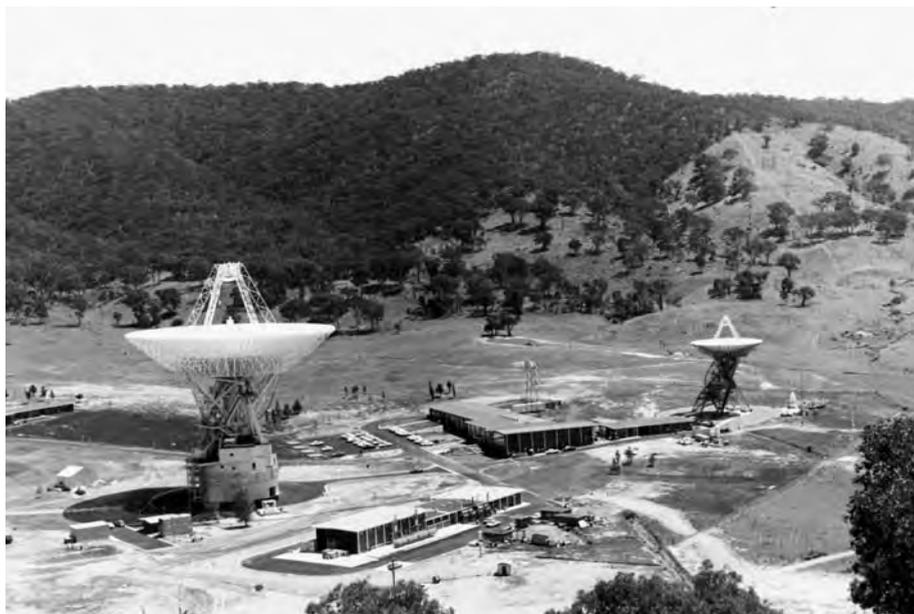
Natural RF shielding from the surrounding hills is evident, as is the size difference between a 64- and 26-meter antenna in this undated photograph of the DSN station at Tidbinbilla. (Unnumbered photograph, Folder 8820, NASA Historical Reference Collection, NASA History Division, NASA Headquarters, Washington, DC)
