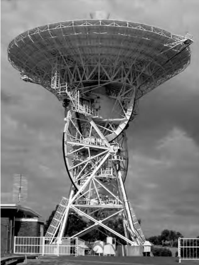
The 85-foot tracking antenna which received signals of mankind's first steps on the Moon on 20 July 1969 still operates today at the Canberra Deep Space Communication Complex in Tidbinbilla, Australia. The antenna was moved from its original Honeysuckle Creek site some 30 kilometers (20 miles) away in 1985. Clearly visible are the two large yokes which allow the antenna to be moved in two "X-Y" axes as it tracks a spacecraft. (Photograph by the author)
