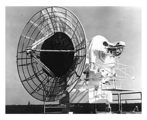
The RCA FPS-16 radar has been widely used at missile ranges since the 1950s. It is a transportable, Single-Object Tracking Radar which operates in the C-band of the electromagnetic spectrum. The photograph shows a FPS-16 at Patrick Air Force Base used in 1961 to track launches out of Cape Canaveral. (Photo courtesy of Patrick Air Force Base Office of History)
