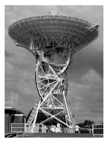
The 85-foot tracking antenna which received signals of mankind's first steps on the Moon on 20 July 1969 still operates today at the Canberra Deep Space Communication Complex in Tidbinbilla. Australia. The antenna was moved from its original Honeysuckle Creek site some 30 kilometers (20 miles) away in 1985. Clearly visible are the two large vokes which allow the antenna to be moved in two "X-Y" axes as it tracks a spacecraft. (Photograph by the author)
