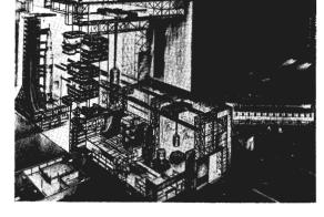
The high and low bay areas of the Vehicle Assembly Building at Kennedy Space Center provided vast space for assembling the Saturn launch vehicles and Apollo spacecraft. At right, the first full-scale Apollo-Saturn V, AS-500-F, rolls out from the VAB on the crawler-transporter May 25, 1966, five years after President Kennedy set a goal of a manned landing on the moon within the decade.
