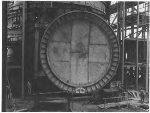
The 56-metric-ton, 11.6-meter-diameter (62-U.S.-ton, 38-foot-diameter) stainless steel door for Chamber A of MSC's Space Environmental Simulation Laboratory was swung into place early in April 1964 to finish enclosing the large test facility. Chamber A was tubular, 35.7 meters high, 19.8 meters in diameter (117 feet high, 65 feet in diameter), and extended 7.3 meters (24 feet) into the ground. It was designed to simulate lunar trips with realism and detail close to those of actual flight.
