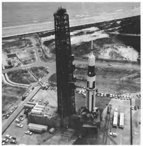
An unusual view of the SA-6 space vehicle was taken from the top of the gantry at Pad 34 during a radio frequency interference test before the launch.
