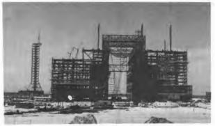
1962 December the Vertical Assembly Building (VAB) at Cape Canaveral. The massive VAB became a space-age hangar, capable of housing four complete Saturn V launch vehicles and Apollo spacecraft where they could be assembled and checked out. The facility would be 158.5 meters (520 feet) high and would cost about \$100 million to build. Subsequently, the Corps of Engineers selected Morrison-Knudson Company, Perini Corp., and Paul Hardeman, Inc., to construct the VAB.
