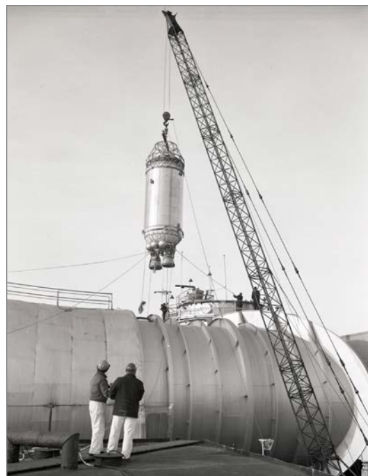
↑ In these two photos from 1964, the Centaur upper stage, equipped with two RL-10 engines, is lowered into the SPC's Chamber Number 1 through its domed hatch. (Photo credit: NASA/GRC/Bill Bowles)
