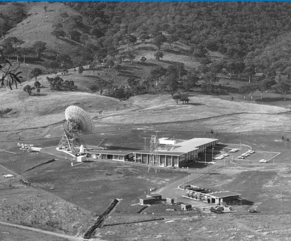
↑ The Tidbinbilla Deep Space Instrumentation Facility is located in the Paddys River valley, about 12 miles (20 kilometers) from Canberra. In this July 1969 photo, a single 26-meter (85-foot) Deep Space Network antenna can be seen next to the facility. (Photo credit: CSIRO/NASA)
