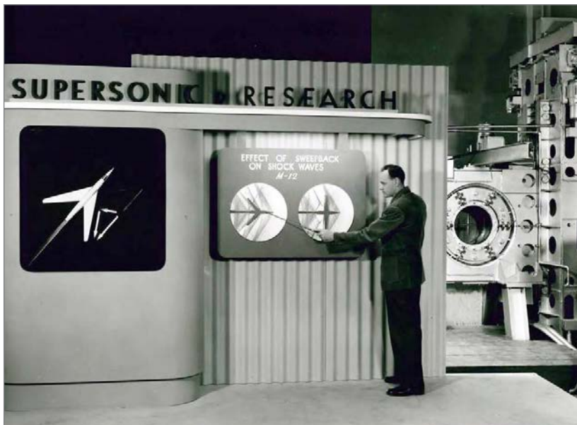
Engineer Walter Vincenti explains the benefits of wing sweep in front of the test section of the 1- by 3-foot supersonic wind tunnel. (Image credit: NASA)
