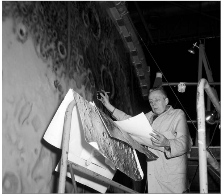
Artists used paintbrushes and airbrushes to recreate the lunar surface on each of the four models comprising the LOLA simulator. (Credit: NASA)
