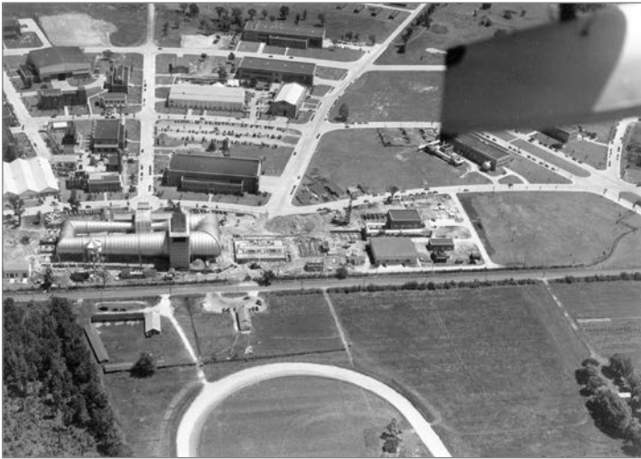
In this photo, the historical building 1195 is in the center of the photo. It is a long, light building with two rows of windows facing a parking lot that still exists. The streets that run along two sides of the building are currently pedestrian walkways. A partial view of the Langley racetrack is visible in the foreground, as is the 16-Foot Transonic Tunnel, which has since been demolished. Across the street from the 16-Foot Transonic Tunnel is building 1148, the Structures and Materials Lab, which is still standing. (Photo credit: NASA)
