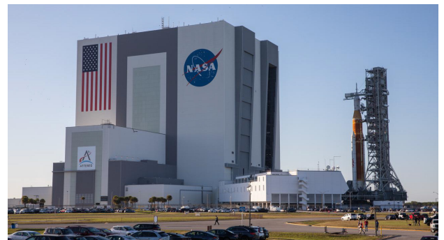
NASA's Space Launch System rocket rolls out of the Vehicle Assembly Building on its journey to the launch pad. (NASA/Kim Shiflett)
