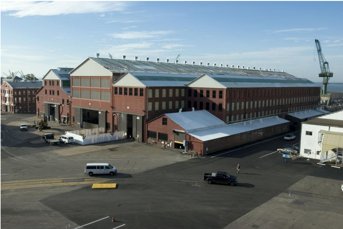
Figure 3. View of the massive 120-year-old machine shop buildings at Northrop Grumman Shipbuilding in Newport News. (Photo courtesy of Northrop Grumman Shipbuilding-Newport News).
