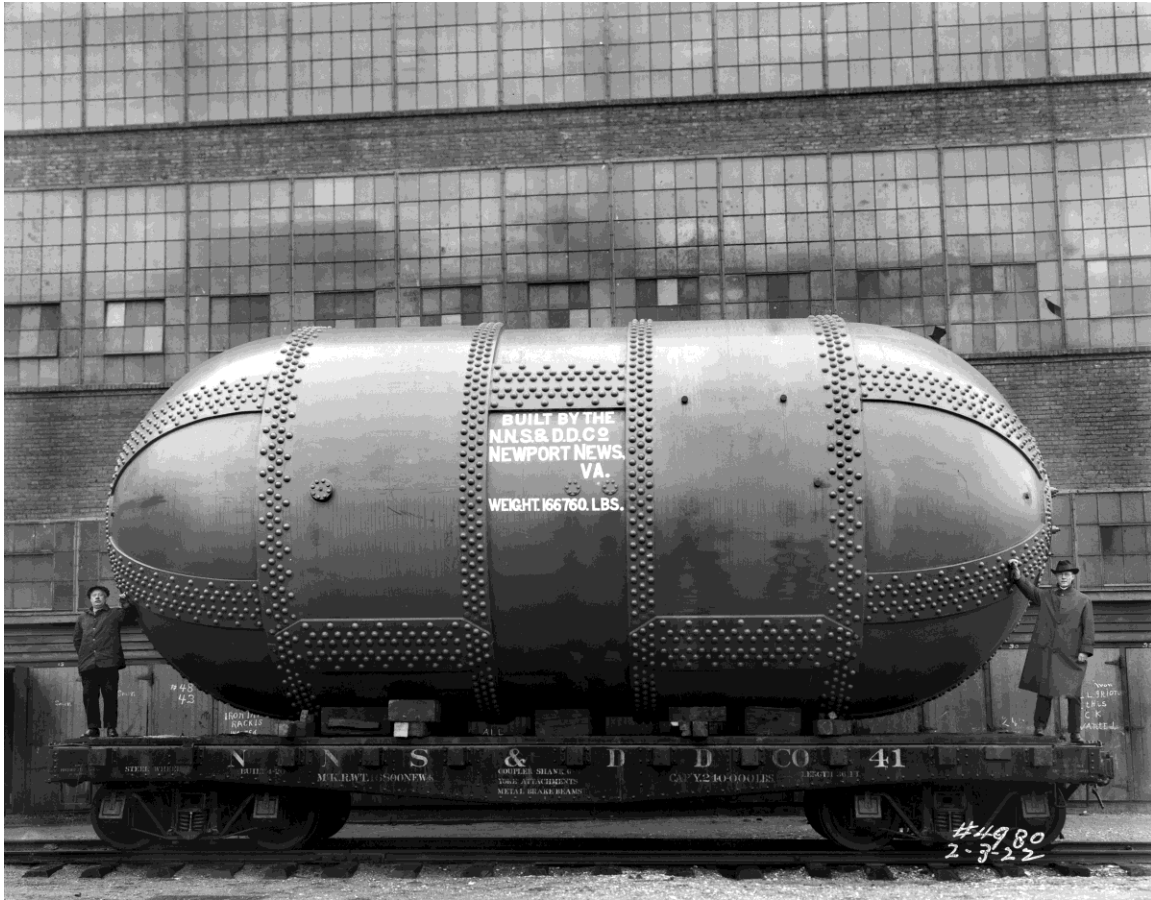
Figure 2. Photograph of the pressure tank of the Variable Density Tunnel at the Newport News Shipbuilding and Dry Dock Company on February 3, 1922. (Photo courtesy of Northrop Grumman Shipbuilding-Newport News).
