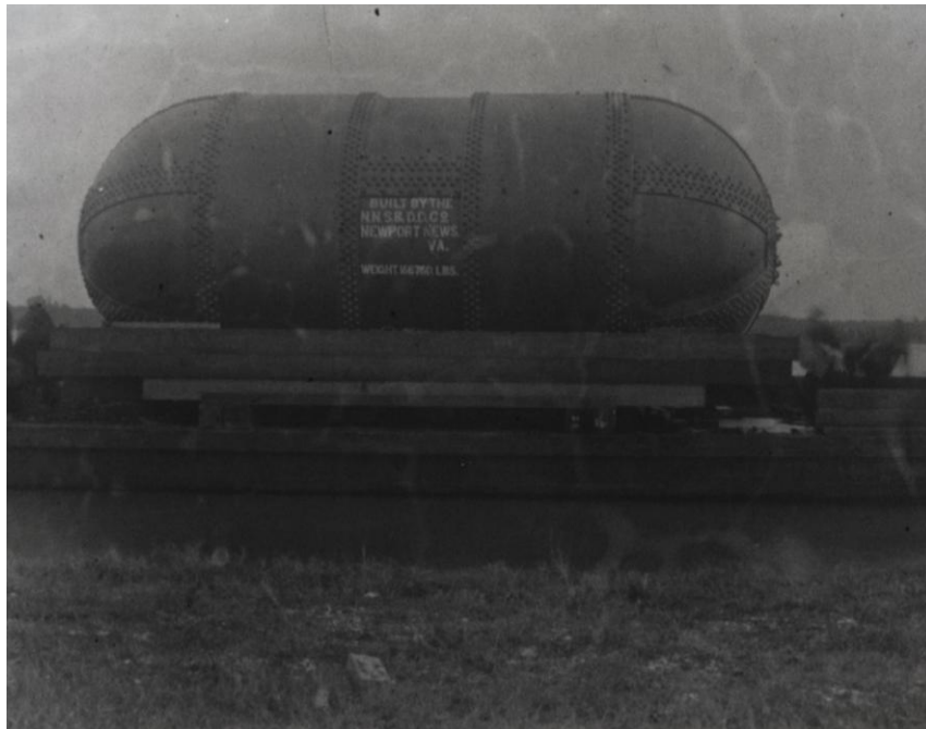
Figure 5. Arrival of the pressure tank of the VDT at Langley via barge in June 1922.
