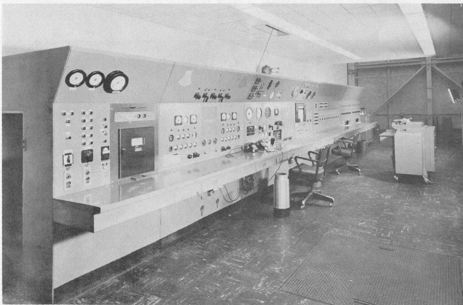
Figure 8.- The control room at the Langley 16-foot transonic tunnel showing data readout equipment at far end of control panel.
