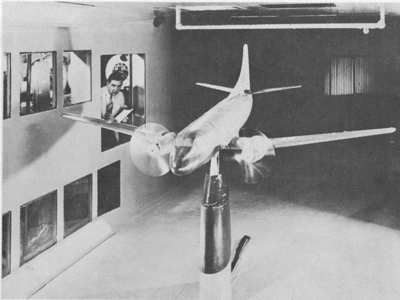
Figure 5.- A single-strut installation of a powered model in the Langley 300-MPH 7- by 10-foot
