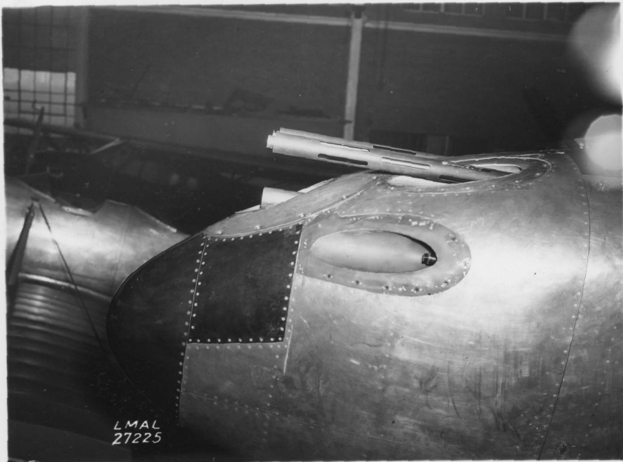
Figure 7. - Armament installation of the YP-38 airplane.
