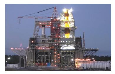
NASA Stennis provides unique facilities for testing SLS RS-25 engines and controllers.
