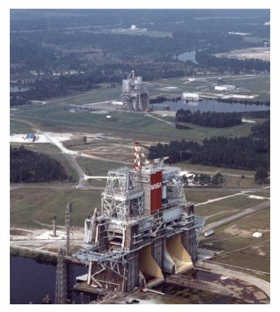
NASA Stennis provides unique facilities for testing SLS RS-25 engines and controllers. The B Complex, foreground, was used for Green Run testing the SLS core stage.
