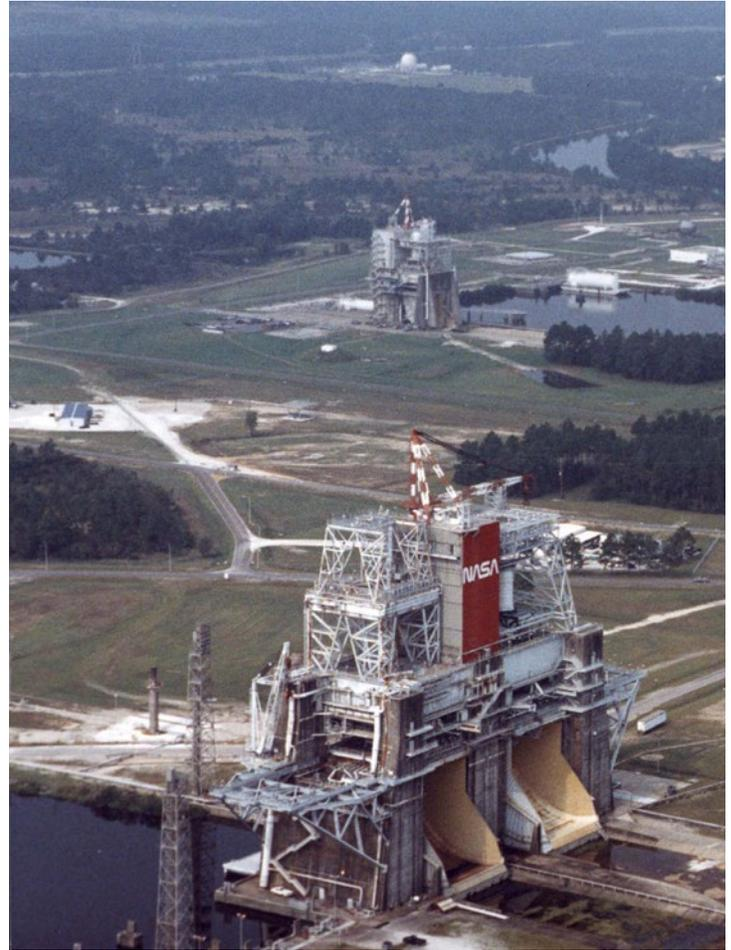
*NASA Stennis provides unique facilities for testing SLS RS-25 engines and controllers. The B Complex, foreground, was used for Green Run testing the SLS core stage.*
