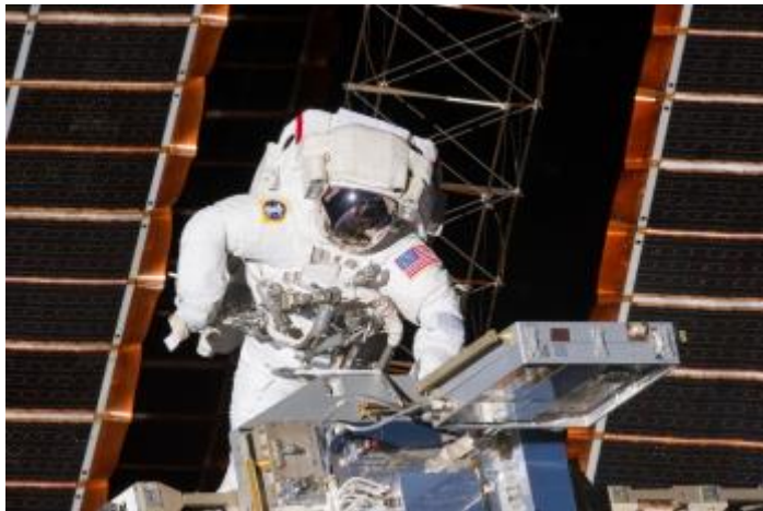
View of STS-134 Mission Specialist Andrew Feustel working to install a new Materials International Space Station Experiment - 8 on the Expedite the Processing of Experiments to Space Station Logistics Carrier 2. NASA image.
