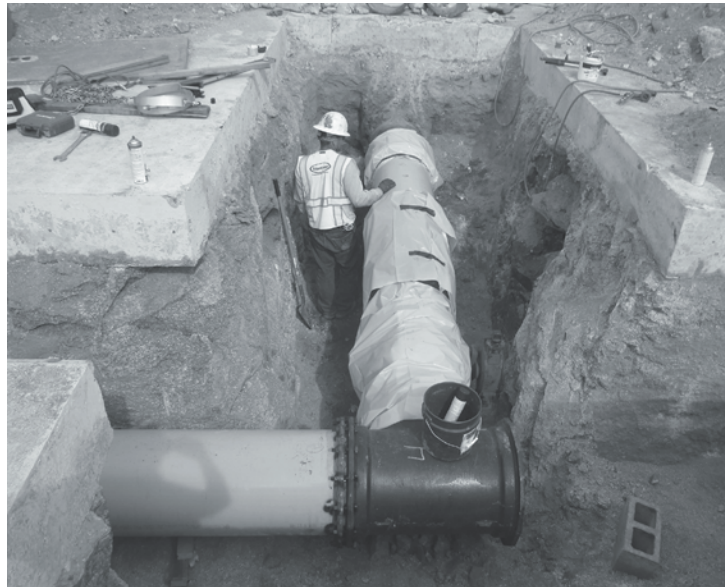
Photo courtesy of Randy Davis of Tony Vacca Construction
