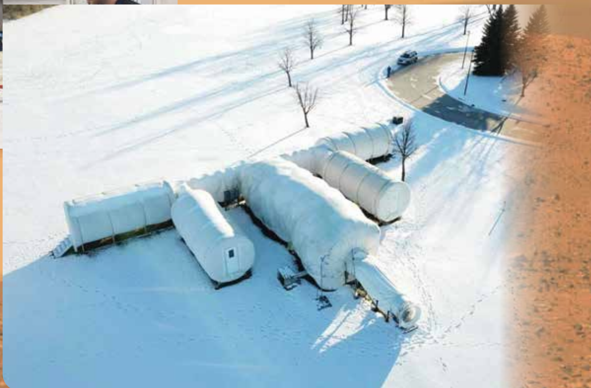
Below: Winter 2018 overview of the completed Lunar Martian Analog Habitat at the University of North Dakota.
