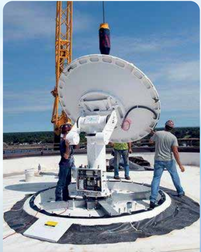
HU: CARE Direct Broadcast Antenna installed on top of the Harbour Centre
