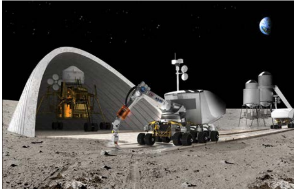
A Contour Crafting robot prints a road in front of a hangar for a lunar lander.
