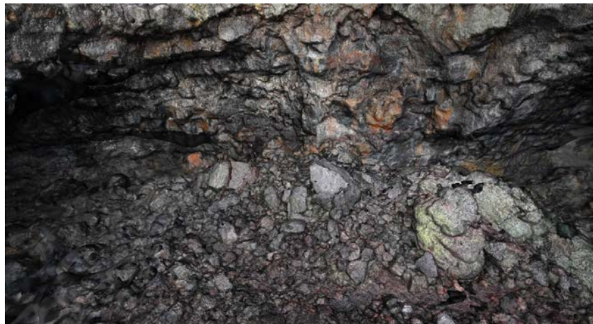
Figure 118: Close-up view of the colorized mesh, showing skylight wall descending to rubble floor.
