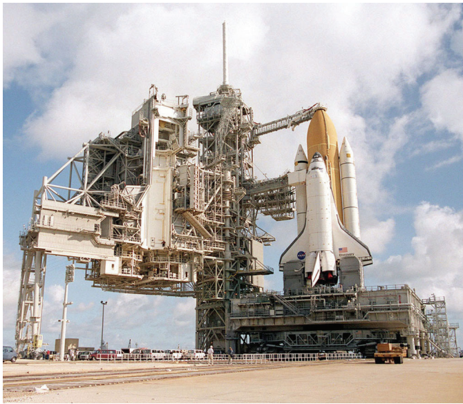
The rotating service structure at left is open to allow Space Shuttle Discovery to roll onto the pad.
