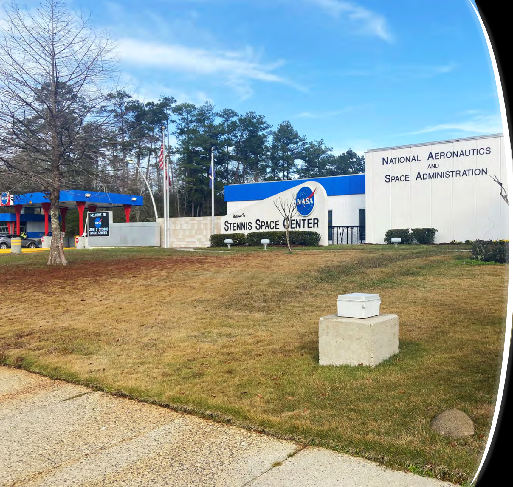
South Gate and Reception Center
