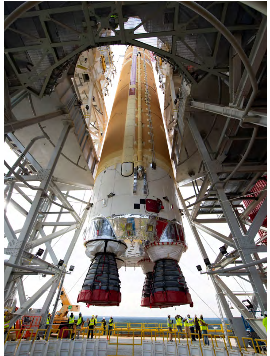
SLS Rocket Installed on the B-2 Test Stand
