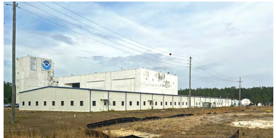
NOAA Warehouse Within the Fee Area at SSC
