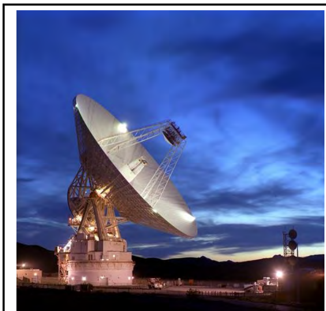
The 70-meter DSS-14 antenna is the largest and most sensitive antenna at the Goldstone Deep Space Communications Complex in California. Operational in 1966 and upgraded in 1998, DSS-14 communicates with deep space missions such as New Horizons, which is on its way to Pluto and Charon. The three Deep Space Network sites- Goldstone; Canberra, Australia; and Madrid, Spain- currently track, receive data from, and transmit commands to over 25 spacecraft, including Voyager 1, which is over 11 billion miles from earth.
