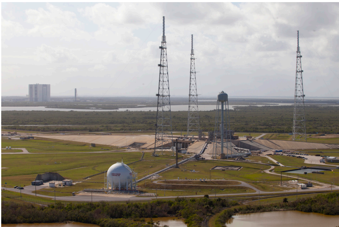
An aerial view of Launch Pad 39B at NASA's Kennedy Space Center in Florida. In view are the three lightning towers. The Vehicle Assembly Building is in view at far left. Photo credit: NASA/Bill White
