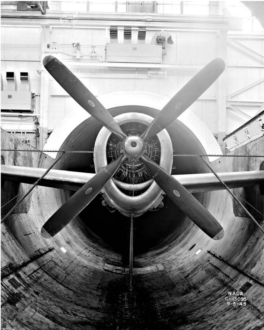
Shown above is a Republic XP-47M Thunderbolt fighter, complete with Hamilton Standard propeller and Pratt & Whitney radial engine, installed in the Altitude Wind Tunnel at the Aircraft Engine Research Laboratory in September 1945. (NACA)
