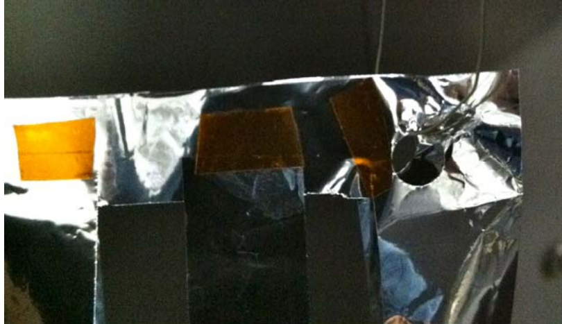
Figure 7.2. Melted membrane from contact with charging wire
