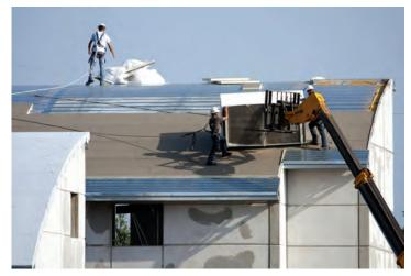
Workers place R-40 rated insulation material on the roof of one of the Propellants North Administrative and Maintenance Facility buildings.
