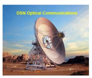
Figure 12.43: Artist overlay of built DSN RF antenna and planned optical segments at its center. Credit: NASA.
