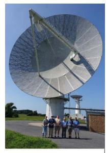
Figure 12.16: 18-meter UHF ground station antenna at NASA Wallops Flight Facility. Credit: NASA.
