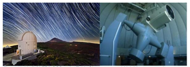
Figure 12.38: (left) ESA-OGS at the Teide Observatory and (right) its 1-meter telescope on an English equatorial mount. Credit: (left) European Space Agency/D. Lopez and (right) European Space Agency.
