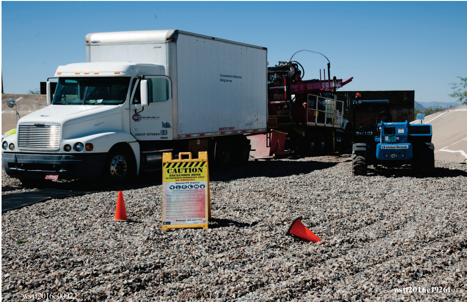
SB-04 (400-EV-131) was the boring/MSVGM well in the northwestern corner of the eastern impoundment. Looking west toward the central berm. Note the Exclusion Zone sign in the foreground.
