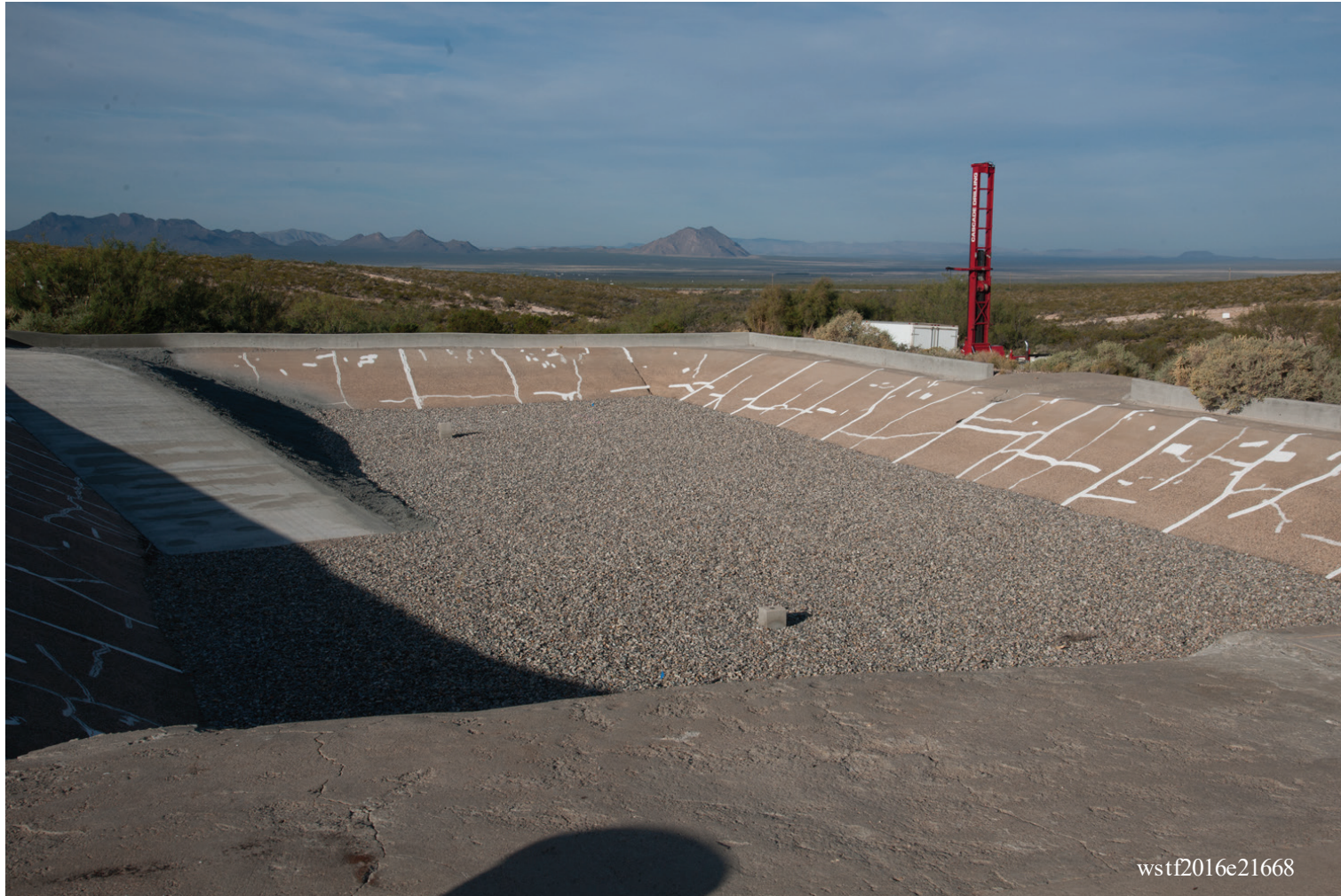
View of the 400 Area Western Impoundment prior to advancing borings SB-07 and SB08. Looking west from the central berm. The drill rig is set up on SB-10, just west of the northwest corner of the impoundment.
