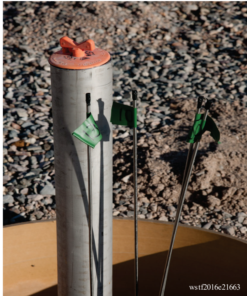
Detail of Well Completion: 400-EV-131
