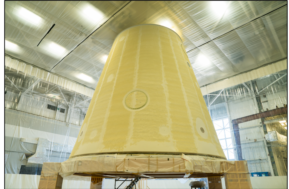
Thermal Insulation Application Complete on LVSA
