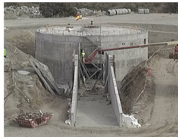
DSS-56 Pedestal Construction
