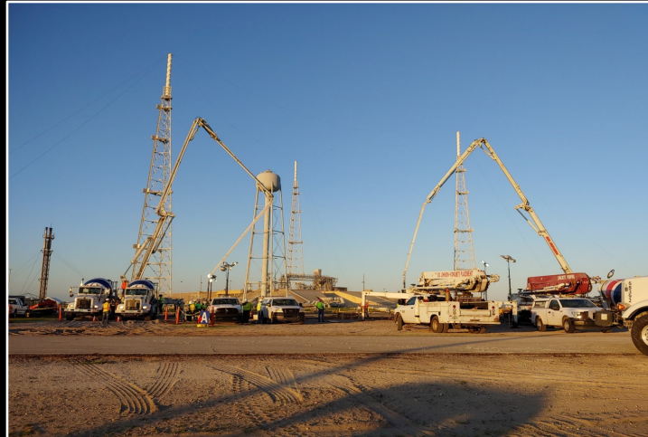
Two concrete pumper trucks pour the foundation to support the new LH2 Dewar at Pad 39B
