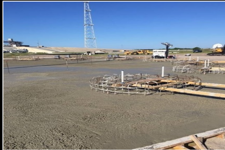
Completion of the LH2 Dewar concrete foundation
