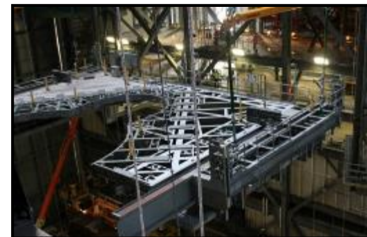
Installing VAB Platform K above HP3
