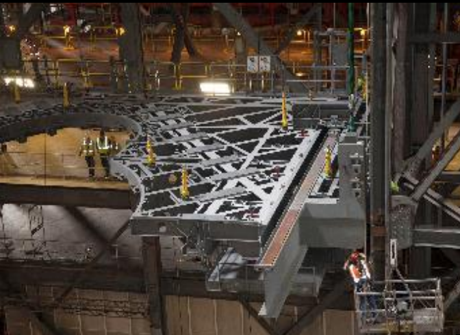
First Work Platform for Space Launch System Installed in VAB
