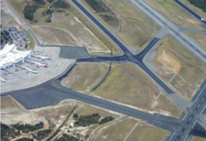
Charlotte-Douglas International Airport.
