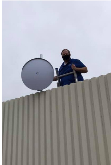
Envoy mounting the network dish to the roof of their building.
