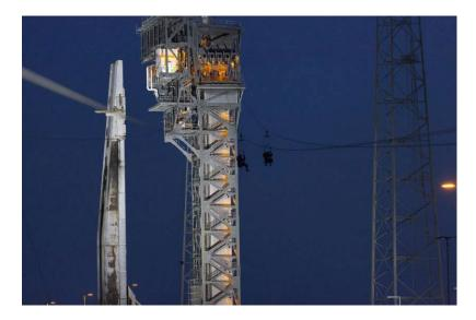
The slide wire emergency escape system features five seats on four separate slide wires, so up to 20 astronauts and ground support personnel can quickly escape from the tower in the unlikely event of a dangerous situation on the launch pad. The egress system allows astronauts and ground personnel to evacuate the Crew Access Tower to a landing zone more than 1,340 feet from the base of the Atlas V, outside of the launch pad perimeter.
