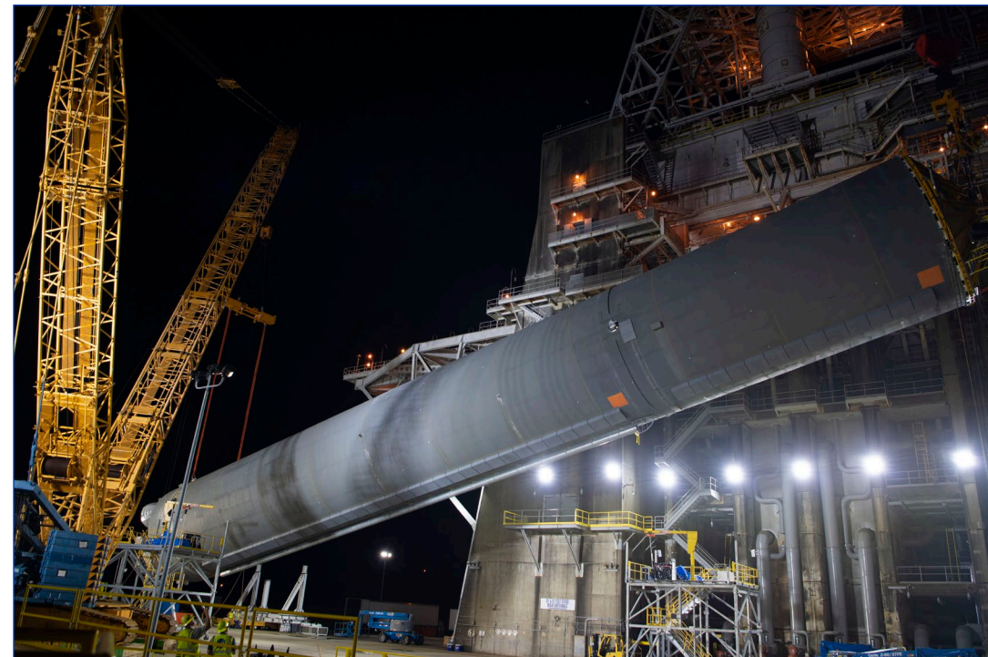
B-2 Test Stand operators perform a lift and installation of the Space Launch System (SLS) core stage pathfinder through the night of Aug. 23-24. The procedure marked yet another milestone as Stennis prepares to install and test the actual core stage that will help power the maiden SLS flight – Artemis I. As photos on this and the following page show, operators used two cranes to lift the pathfinder from its horizontal position, “break” it over into a vertical position and hoist it up and into place on the stand. The exercise allowed operators to practice the procedure and helped confirm the test facility is ready to receive the core stage when it is delivered later this year.
