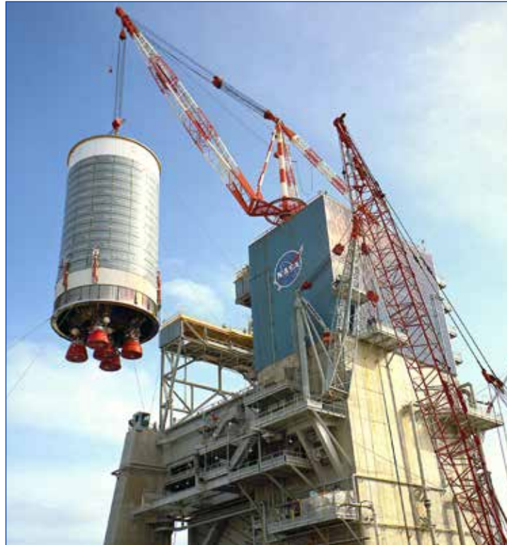
The Saturn S-II-T “T-Bird” rocket stage is lifted onto the A-2 Test Stand at the then-Mississippi Test Facility in October 1965 in preparation for test firing.
