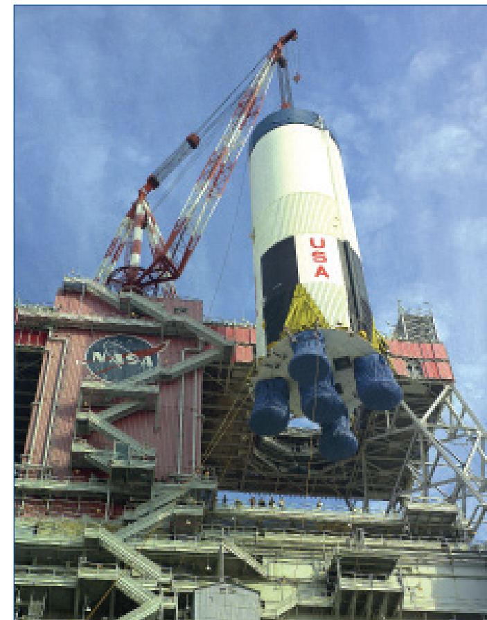
A Saturn V S-IC stage is hoisted into place during Apollo testing. First and second stages of Saturn V rockets were tested at Stennis prior to launch.
