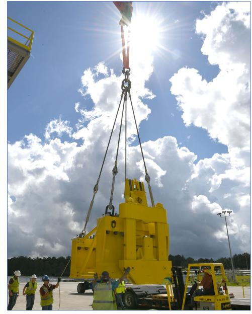
B-2 Test Stand team members prepare to lift one of two so-called "yellow boxes" onto the stand for installation. The yellow boxes will help anchor NASA's Space Launch System core stage in place during testing.
