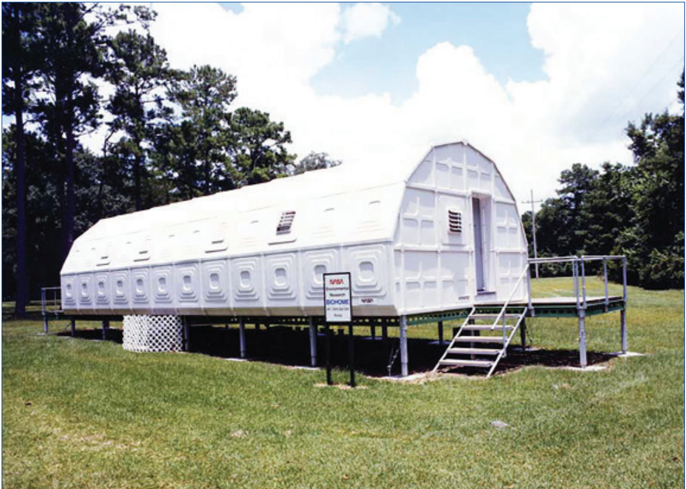
In the 1980s, the BioHome at NASA's Stennis Space Center was 45 feet long, 16 feet wide, and used common indoor house plants as living air purifiers.
