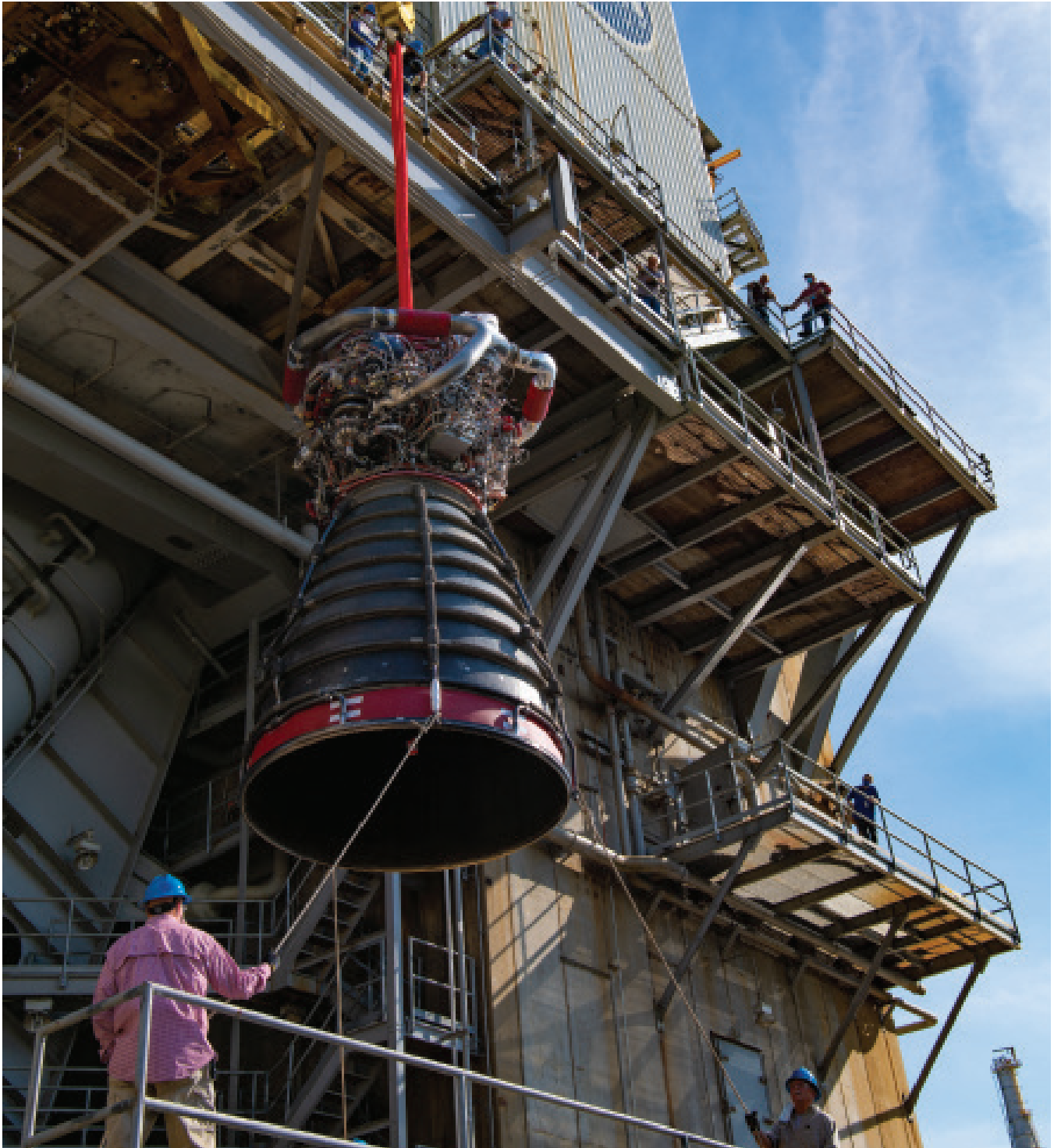
RS-25 developmental engine No. 0525 is raised onto the A-1 Test Stand at Stennis Space Center on Nov. 3, 2021. See page 4 for more.
