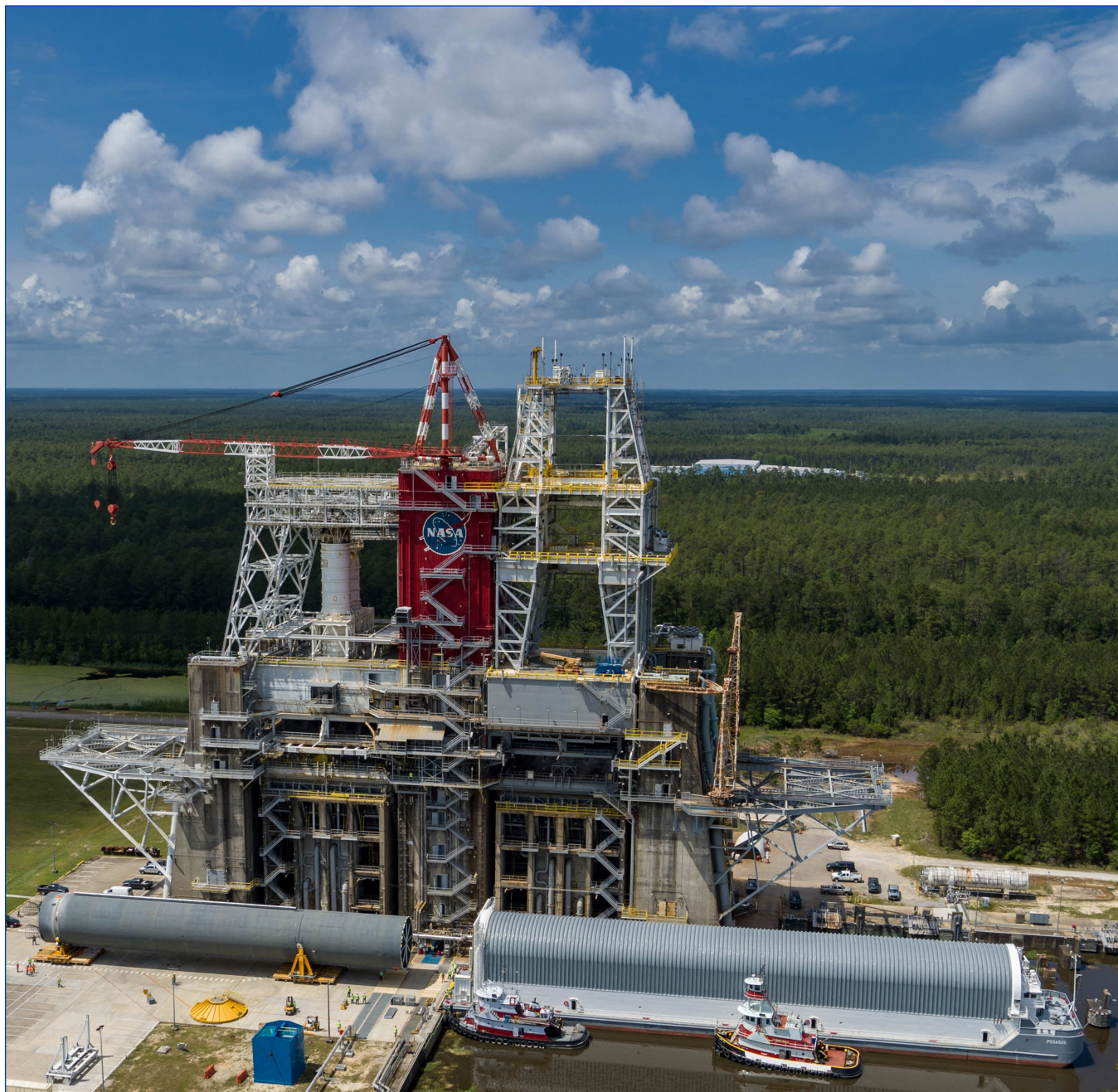
The Space Launch System (SLS) core stage Pathfinder – a replica of the actual core stage – sits on the B-2 Test Stand tarmac at NASA's Stennis Space Center after it was rolled out of the Pegasus barge May 3. Stennis will use the Pathfinder to confirm all is ready for arrival of the actual SLS flight core stage, which will be tested prior to its launch on Exploration Mission-1. See page 3.
