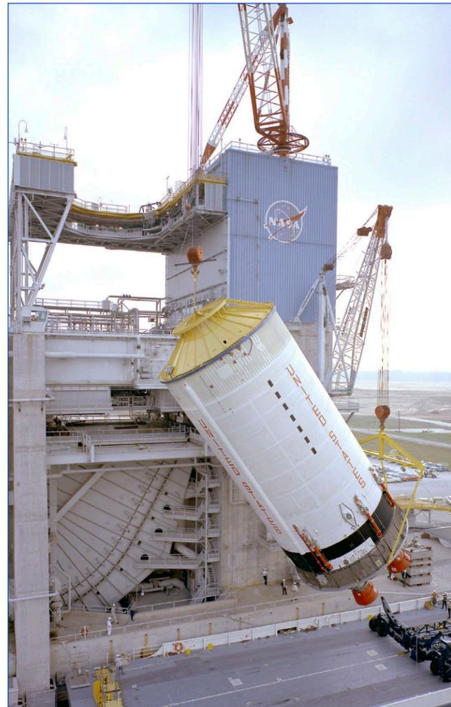
(Above photo) A Saturn V second stage rocket is lifted into place on the A-2 Test Stand at Stennis Space Center for Apollo Program testing in the 1960s.
