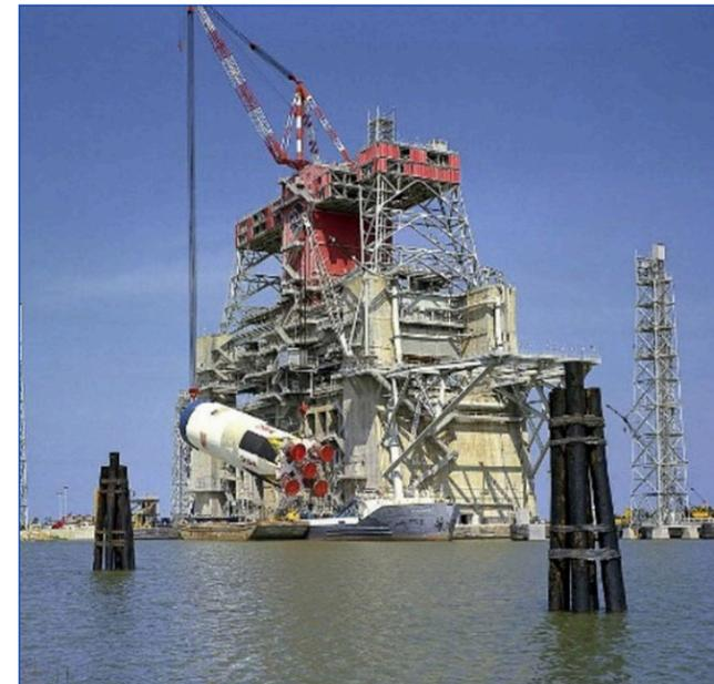
(Top center photo) A Saturn V first stage is lifted into place on the B-1/B-2 Test Stand at Stennis Space Center for Apollo Program testing.
